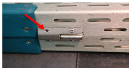
Fractured/missing rivet
